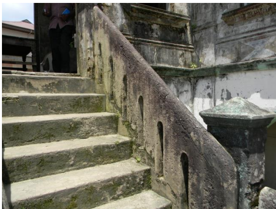
Figure 13: Ornamented staircase Source: Author (2022)
