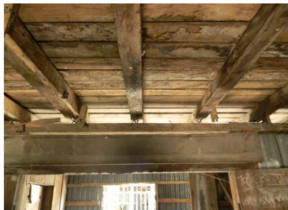
Figure 9: suspended timber floor Bobmanuel house Abonema Source: Author (2016)
