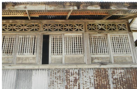
Figure 7: Example of Portuguese timber fretwork Source: Author (2022)
