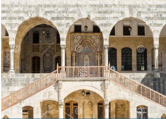
Figure 20: A typical Lebanese Villa with a grand double-sided staircase to a main first floor entrance
