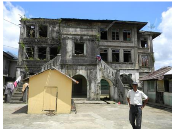
Figure 22: double-sided staircase to upper floor entrance
