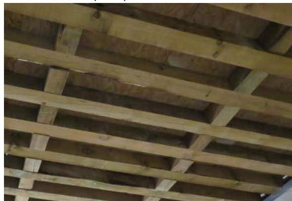
Figure 8: Restored suspended timber floor Source: House in Lisbon, Henriques (2020)
